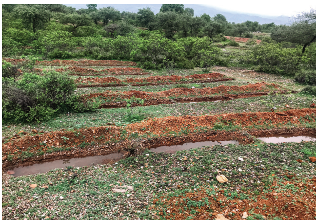
CCT (Continuous Contour Trench) one of the most popular and effective SWC treatment
