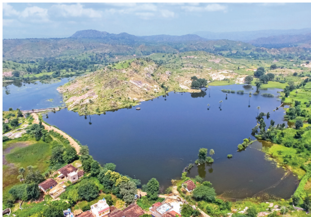
Mandili water conservation- Rejuvenated the defunct existing Anicut in Dayli Village
