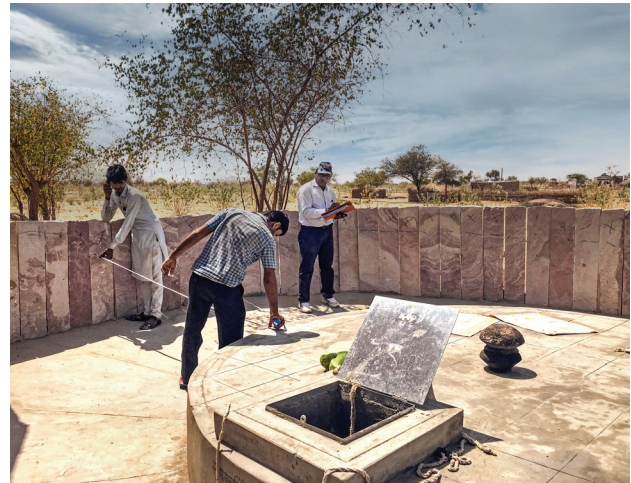
The pakka tanka post construction
