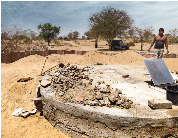
The pakka tanka during construction
